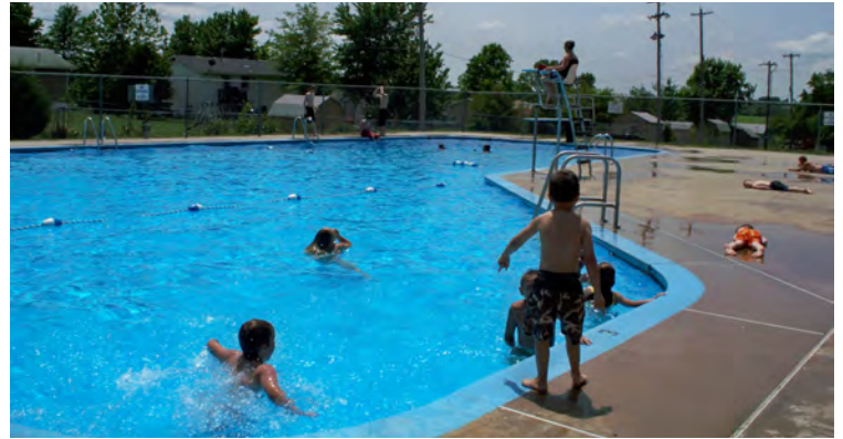
The Carbondale city pool was recently renovated.
