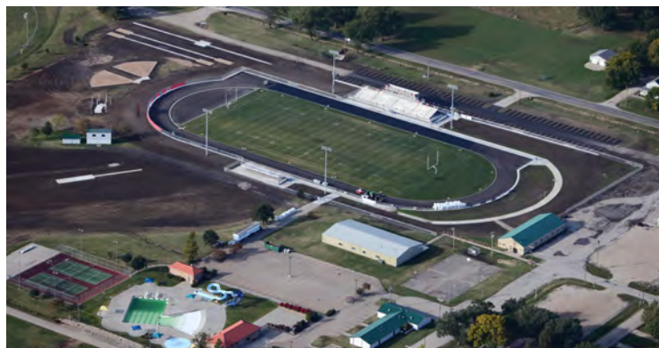
The recently rebuilt USD 420 sports complex at Jones Park.
