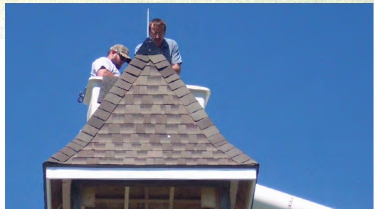
Volunteers replace the roof of the schoolhouse in 2016.
